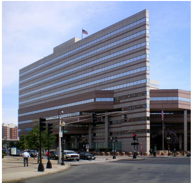
The 600,000sf Thomas P. O'Neill, Jr. Federal Building in Boston, MA uses the Niagara 4 open framework as its BAS. This Energy Star rated and LEED Platinum Certified facility houses various government agencies.
